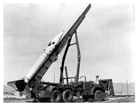
Honest John rocket on launcher. Courtesy, U.S. Army Aviation and Missile Life Cycle Management Command.
