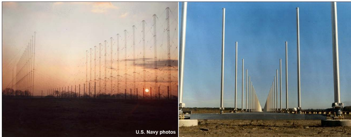
Figure 15. ROTHR Sites: Transmit (left) and Receive (right)
