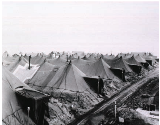
May 8, 1944, Anzio, Italy: The sides of the ward tents of the 94th Evacuation Hospital were reinforced with earthworks.
