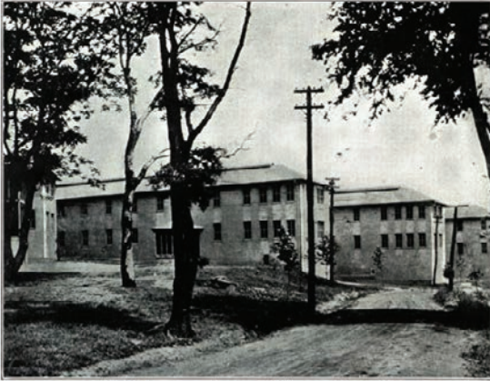
FIG. 192.—Two-story wards constructed of tile. General Hospital No. 2.
