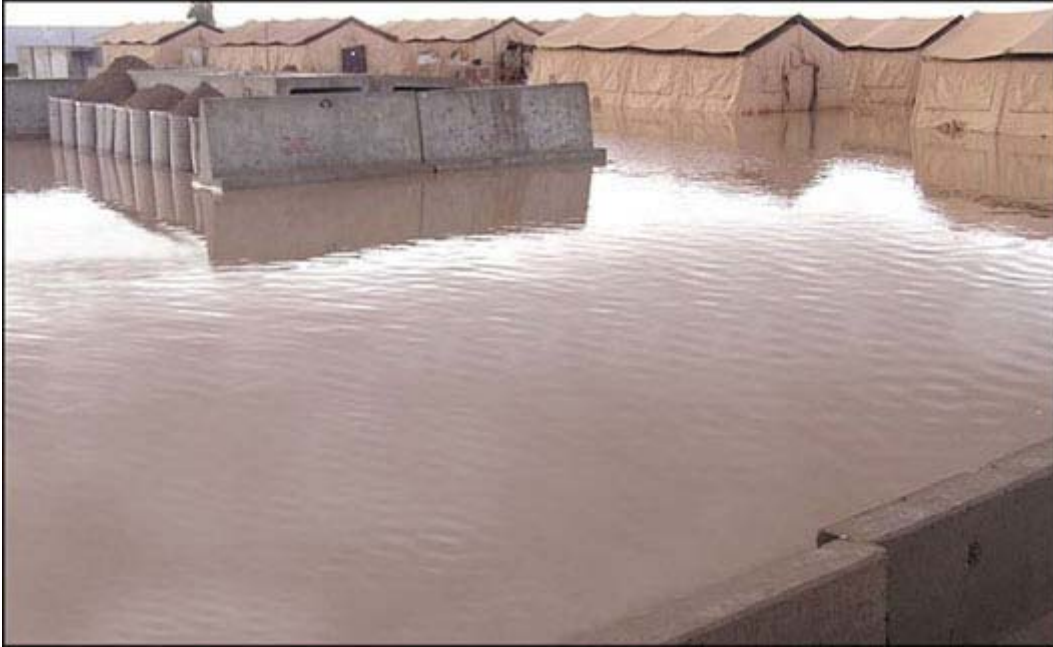
In 2004, Kirkuk Air Base, Iraq, received nearly two inches of rain overnight leaving many areas of the base, including living areas for Airmen and Soldiers, deluged by water. Although constructed on relatively flat terrain, extensive drainage structures, including ditches, were not accounted for in the design plan. This could have mitigated the effects of overwhelming rainfall and flooding around the base.
